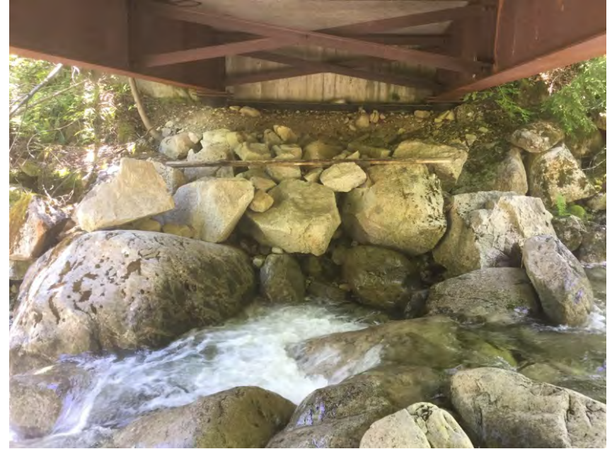
Right Bank Abutment when facing downstream
