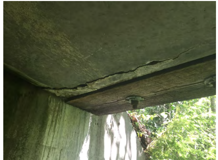
Downstream left approach deck panel
