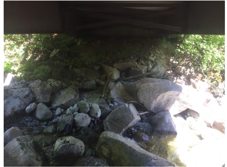
Left Bank Abutment when facing downstream
